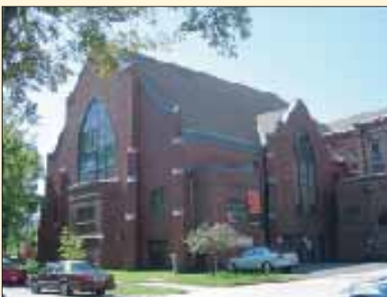
from Aldrich looking southwest
